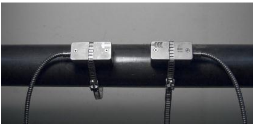
Illustration 7: Sensor mounting with tension straps and clamps
